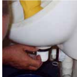
Insert and fix new fitting
