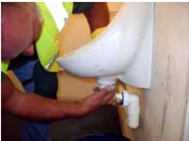
Remove trap/U bend from urinal
