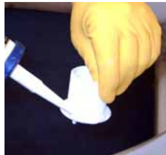
Apply Sealant to fitting
